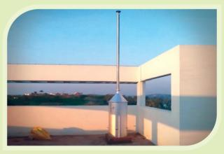
Burning Capacity Chamber Size in mm Chimney size Pipeline 30 kg 700 x 1250 3 metre 6" SS 304 grade
